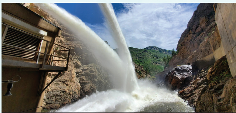
Water cascades from Strontia Springs Dam, located six miles up Waterton Canyon southwest of the metro area, into the South Platte River, one of two major river systems in Denver Water's collection system. (Photo: Denver Water)
