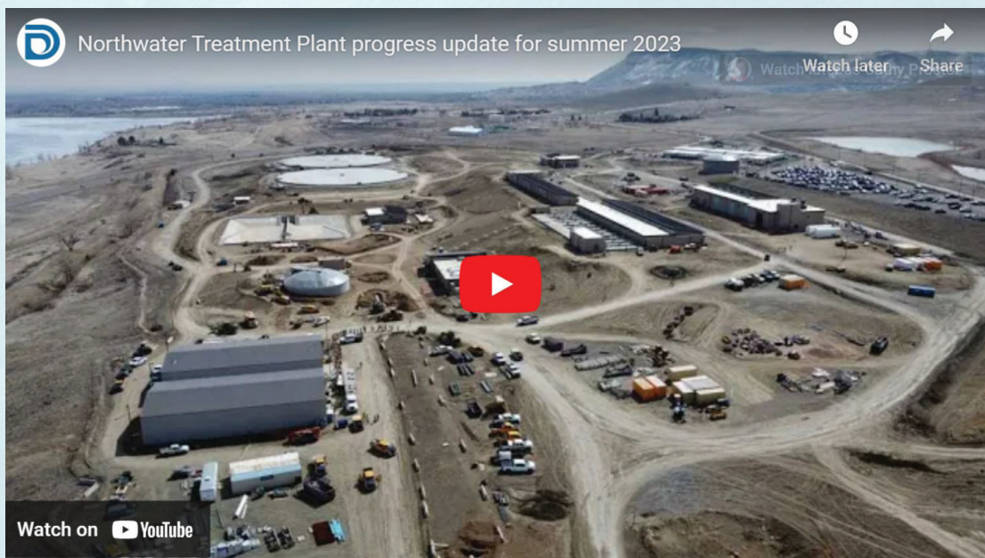
Video: Northwater Treatment Plant progress update for Summer 2023.
