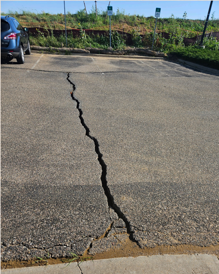
Ongoing parking lot repairs. (Photo: Arapahoe County)
